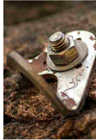
Figure 8. Bolt and bolt hanger.
